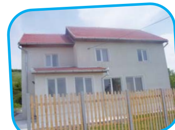
Emergency Housing Unit - After
